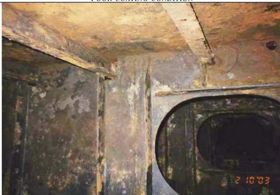
POOR COATING CONDITION
