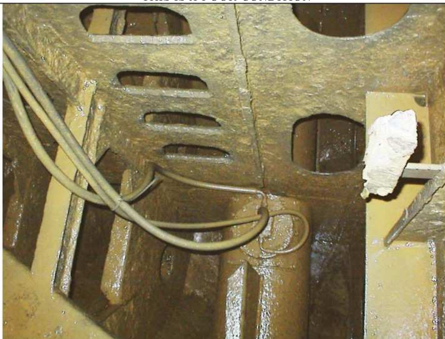
TRANSITION FAIR TO POOR COATING CONDITION: THIS IS A POOR CONDITION
