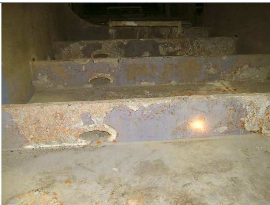
TRANSITION FAIR TO POOR COATING CONDITION: THIS IS A POOR CONDITION
