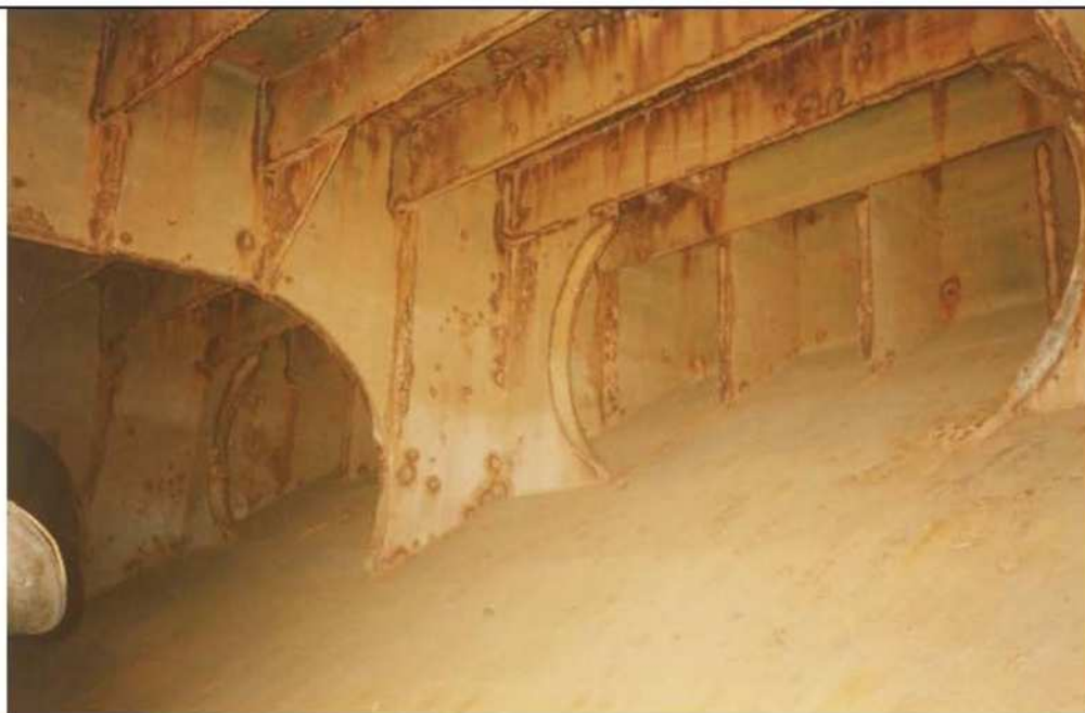
TRANSITION FAIR TO POOR COATING CONDITION: THIS IS A POOR CONDITION
