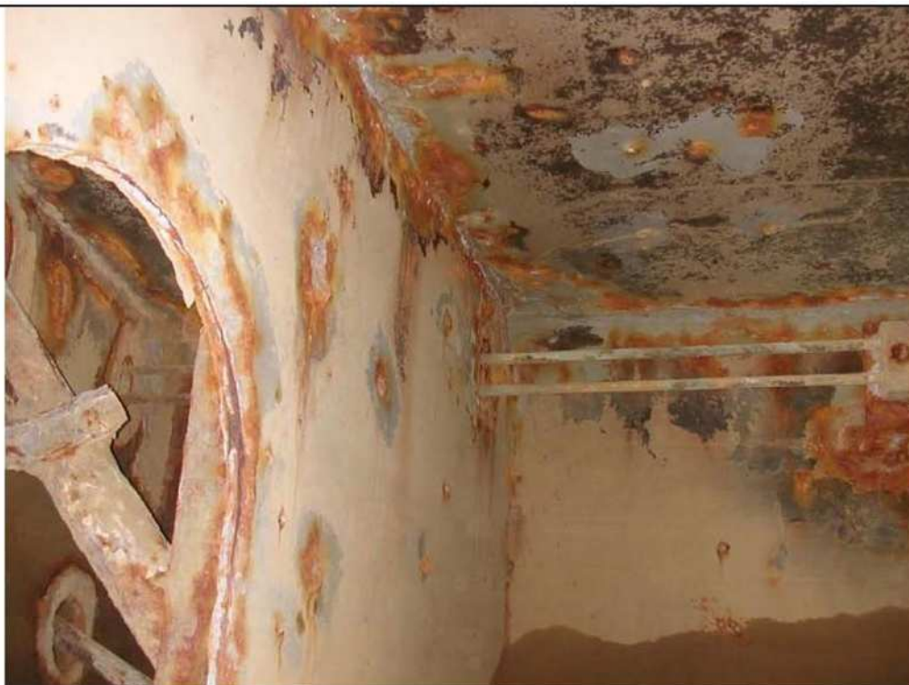
TRANSITION FAIR TO POOR COATING CONDITION: THIS IS A POOR CONDITION
