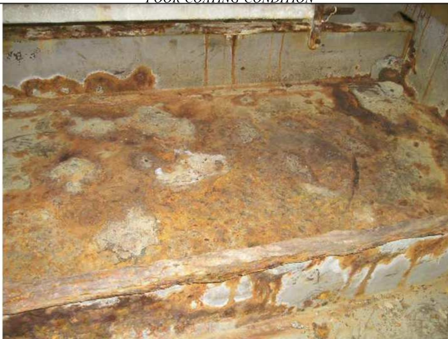
POOR COATING CONDITION
