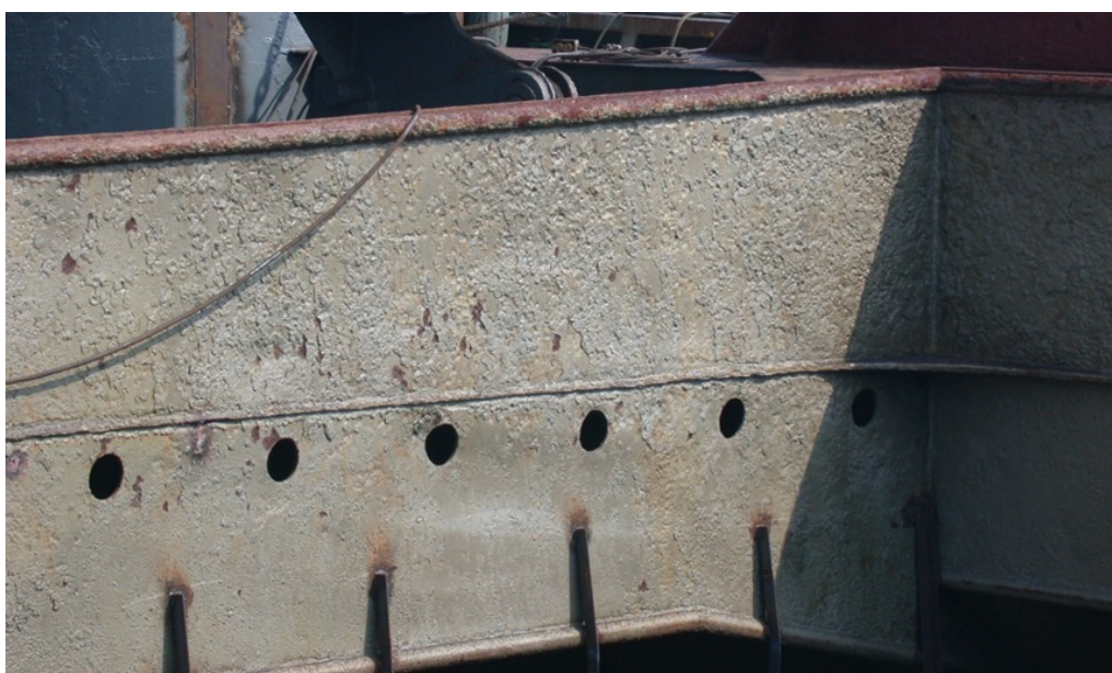
Photograph 1 Heavy corrosion of hatch coaming
